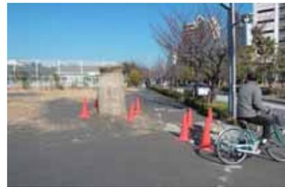
Uplifted manhole by liquefaction
