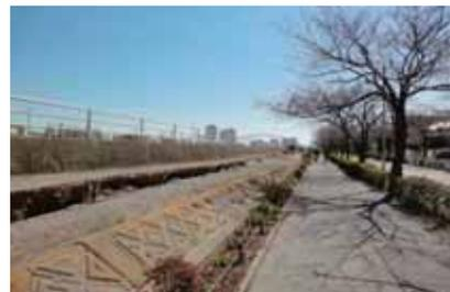
Bumped seawall caused by liquefaction
