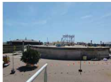
Picture.2: Glenelg Wastewater Treatment Plant
