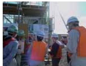
CTI Members showing us reconstruction works in Sendai
