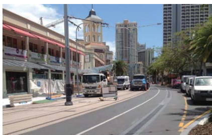
Construction Site of Gold Coast LRT
