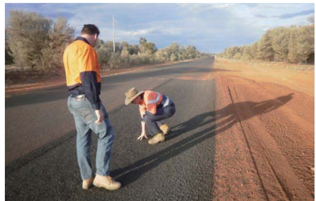
Photo 3-1 Checking the construction site
