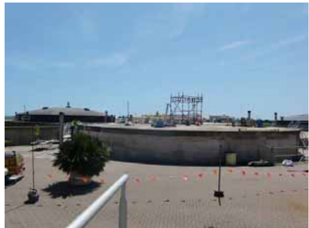
写真 1:Glenelg Wastewater Treatment Plant
