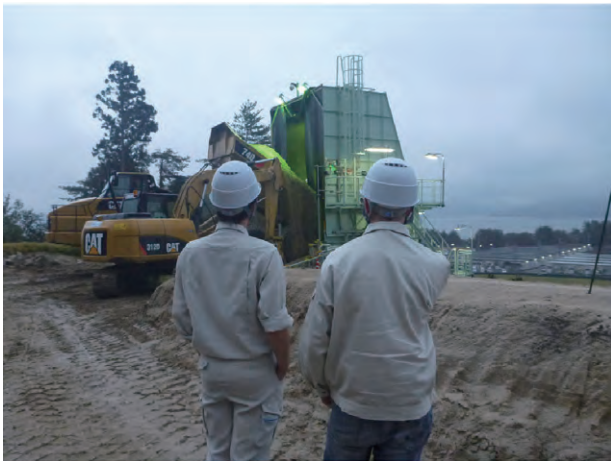
Photo 2: Inspecting earth moving escalator
