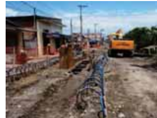
Sewer Improvement Project
