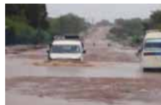
Culvert No.14 - Flooded during heavy rain (Before the Project)
