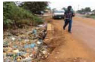
Munuki Bridge - Overflow during heavy rain (Before the Project)
