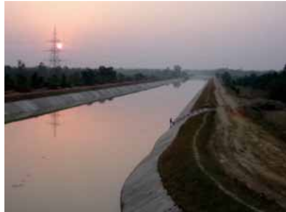
Main Canal, Rengali Irrigation Sub-Project (L.B.C-II, Phase-I), India, with JICA Loan
