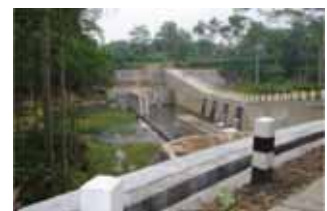
Sabo Dam in Putih River (PU-RD5)
