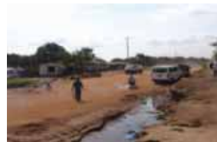
Culvert No.13 - Flooded during heavy rain (Before the Project)
