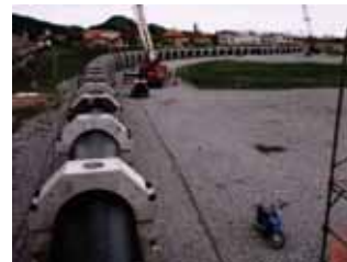
Water Development Project
