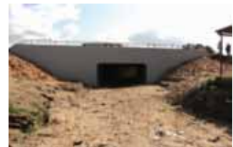
Culvert No.13 - After Completion
