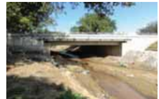
Korbou Bridge (No.9) - After Completion
