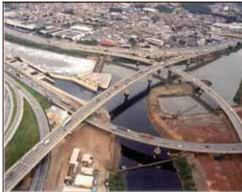
Environmental Improvement Project
