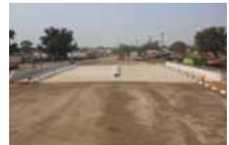
Mudarat Bridge (No.6) - After Completion
