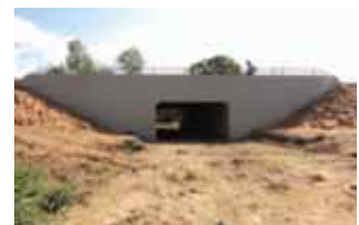
Culvert No.14 - After Completion
