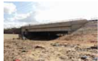
Munuki Bridge (No.12) - After Completion
