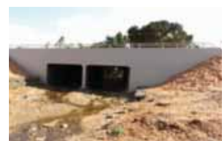
Culvert No.15 - After Completion
