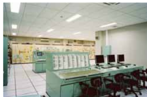
Engine Room Simulator: BP3IP
