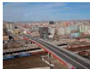
Fly-over section above Ulaanbaatar Railway
