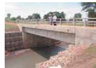
Section 1, Atiabar Bridge
