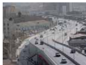
Southern approach road (view from north to south)
