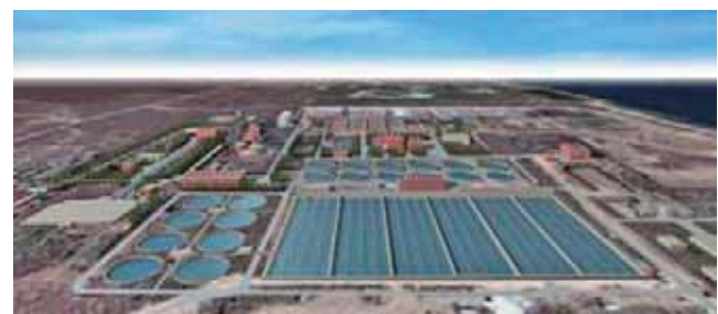
Sewerage Treatment Plant
