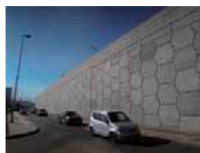
Reinforced earth retaining wall for approach roads
