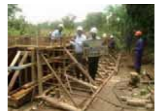
Precast girder work on-the-Job training for District staffs (Soft Component)
