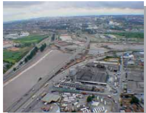
ODA Loan Project Teite river basin depollution Project in Brazil
