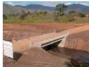
Section 2, Aringa Bridge L=15m
