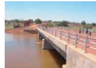
Section 4, Otaka Bridge L=45m
