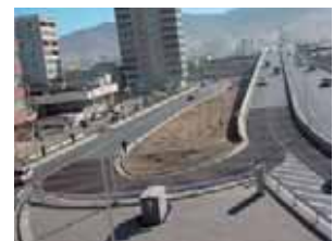
Northern approach road (view from north to south)
