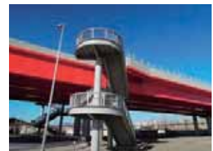
Staircase at east-south portion of fly-over section
