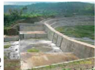
Groundsill and Revetment on Batan River
