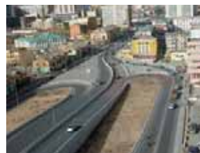
Northern approach road (view from south to north)
