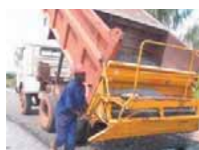
Section 6, DBST work, chips sprayer
