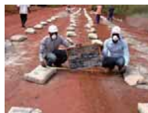
Section 6, Cement stabilization work
