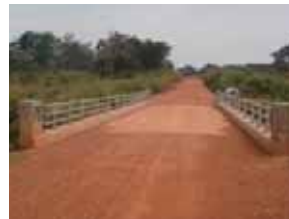
Section 3, Ayago Bridge L=15m
