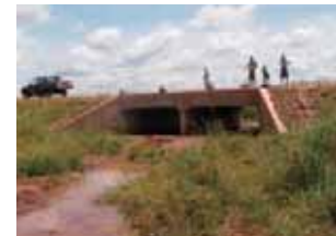
Section 1, Box culvert
