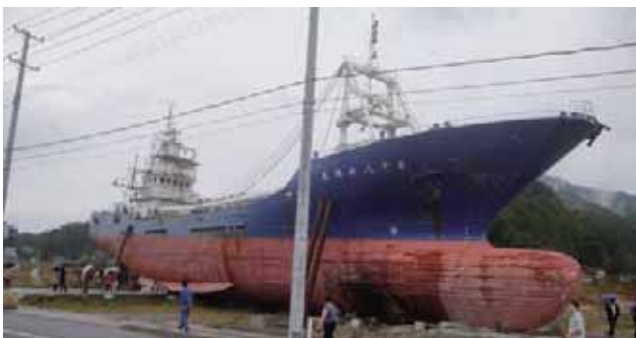
Stranded ship in Kesennuma City
