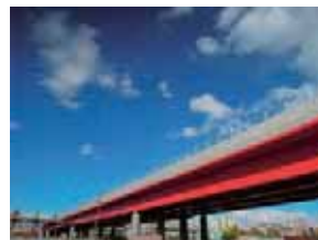
Fly-over section between Railway and Narny Zam
