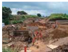
Section 2, Aringa bridge (during construction)
