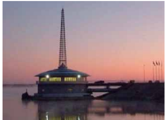
Water Intake Pump Station
