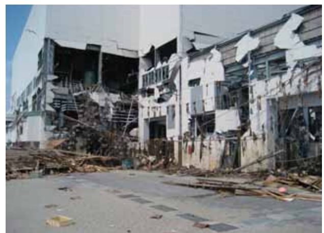
Sewage treatment facility tangled by fish nets Photo: Nihon Suido Consultants
