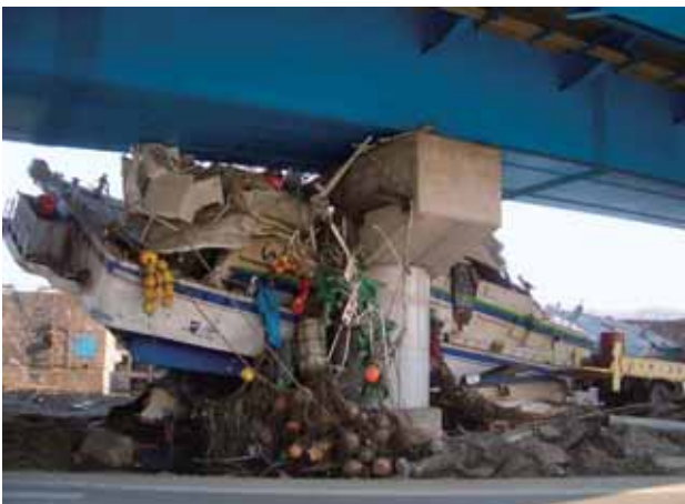
Ship drifted by Tsunami was trapped by bridge pier
