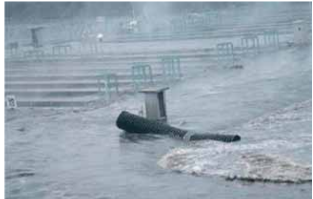
Flooded sewage treatment facility Photo: Tokyo Engineering Consultants
