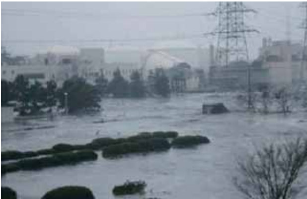
Site of flooded sewage treatment Facility
