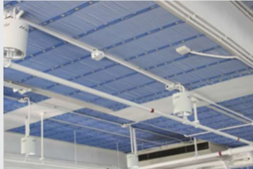
Radiant ceiling cooling system by capillary tubes
